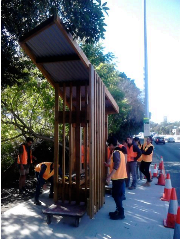
Figure 16: Bus shelter installation on site
