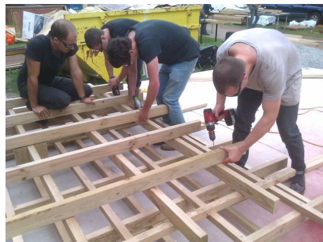
Figure 7: Prefabricating a prototype roof element in the ALVA workshop.
