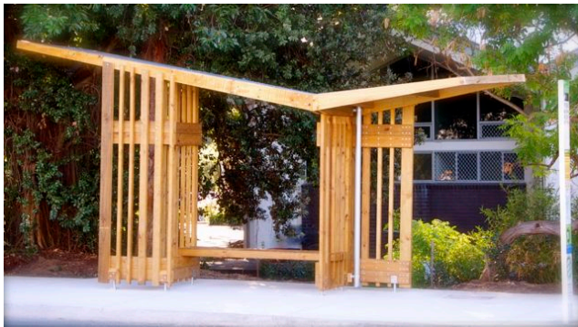
Figure 17: The completed bus shelter
