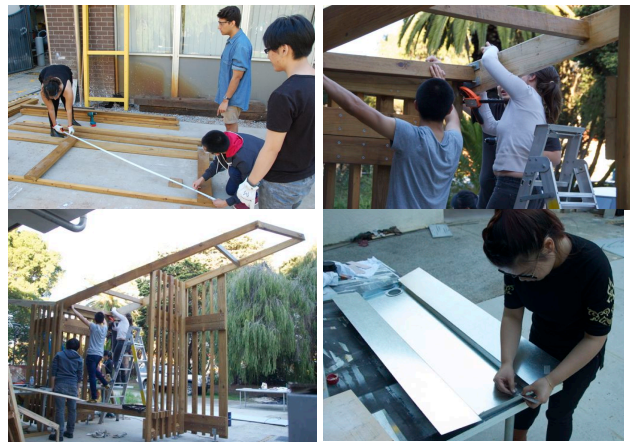
Figure 15: Bus shelter under construction in the ALVA workshop.
