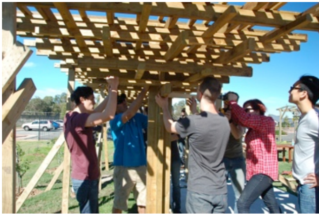
Figure 8: Students installing one of the roof elements on site
