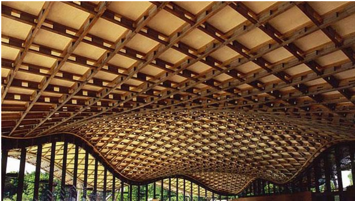
Saville Garden Grid shell. Images: Green Oak Carpentry
