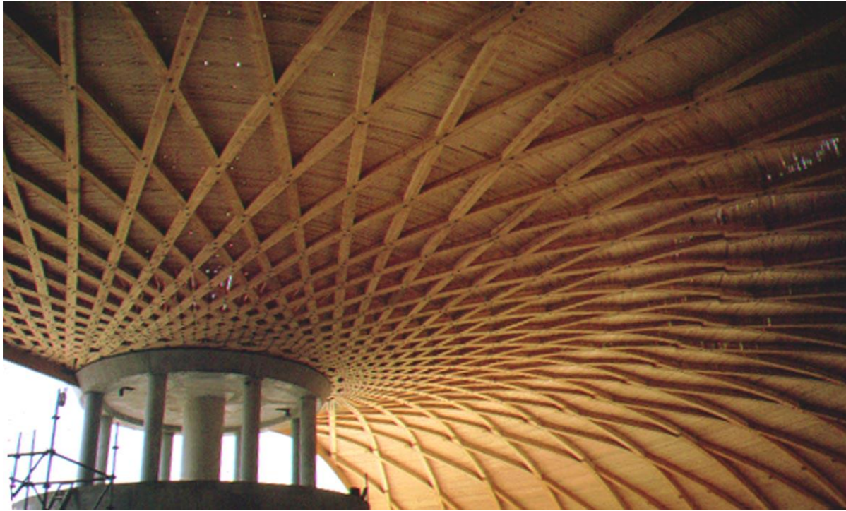
Grid Toroidal roof. St Quentin, Paris. Images: Michael Flach
