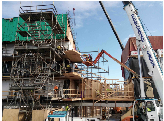
Figure 4: CLT being installed on site.
