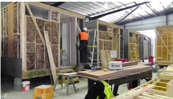
Figure 3: Modules under construction in the factory.
