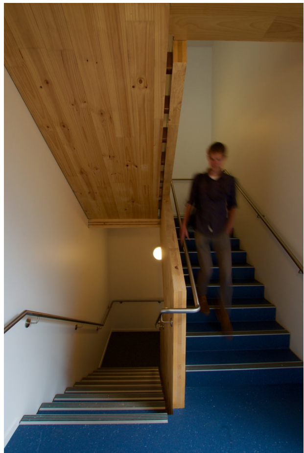
Figure 5: CLT expressed in the stairwells.
