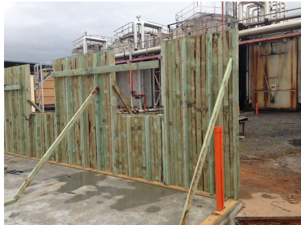
Figure 11: Panels positioned and temporarily propped
