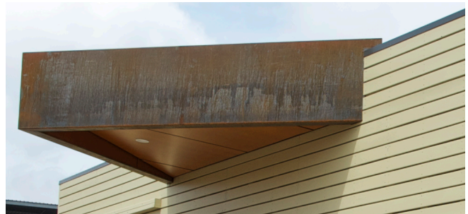
Figure 15: Portico angled at 45 degrees and clad with Corten weathering steel
