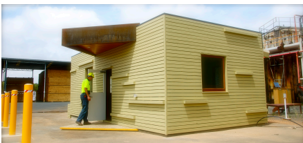
Figure 1: The completed Wespine Kiln Control Facility
