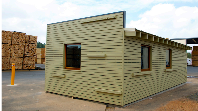
Figure 15: The completed building. The images show the feature horizontal cladding elements. The kilns and stacked timber are in the background.
