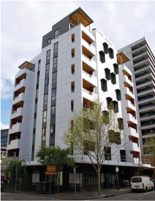
Figure 1.19 - Forté Building. - Photo - D.Bylund
