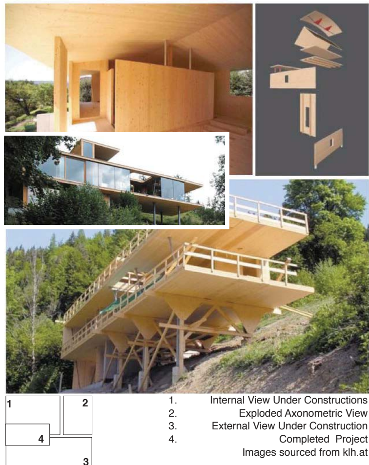
Figure 1.40 CLT projects and exploded panel view. Images supplied by KLH
