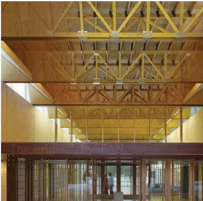
Figure 1.26 Large scale nail plate trusses. Image supplied by Carter Holt Harvey
