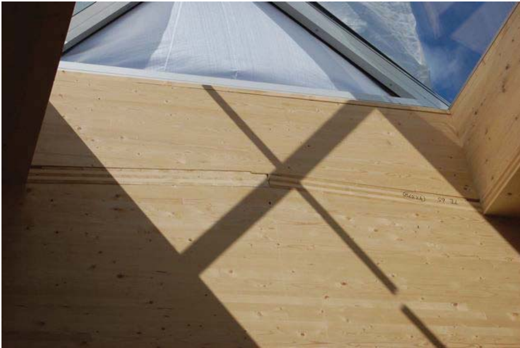
Figure 2.27 Detail of CLT building under construction in Sweden. Photo. D.Bylund
