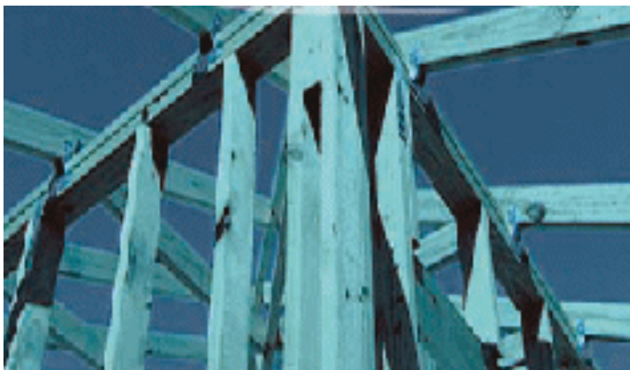
Figure 2.16 Image of Wespine's Blue Pine in a typical stick wall frame application. Image sourced from wespine.com.au
