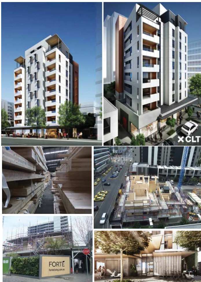
Figure 1.29 Forté Apartments artist impression and under construction.
