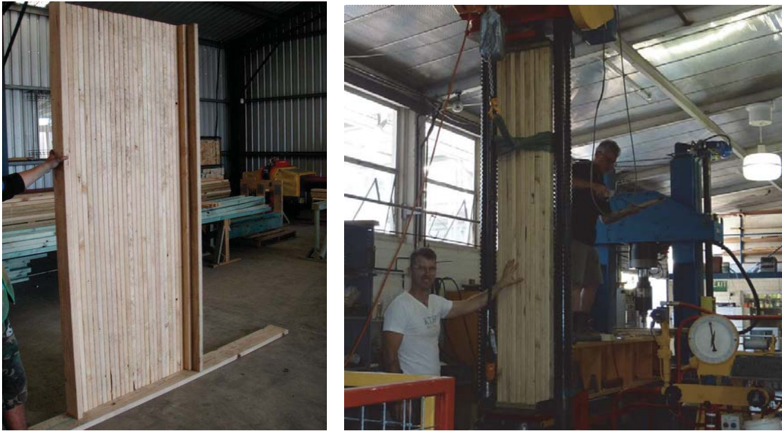
Figure 2.6 Prototype panel being prepared for load testing at UWA's Civil Engineering physical testing facilities.. Full scale prototype under construction (left) and completed (right).
