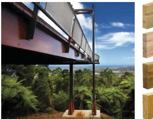
Figure 1.24 Observation platform, material supplied by Hyne Timber and detail of beam products. Information and images sourced from the authors's interviews with Hyne management and hyne.com.au.
